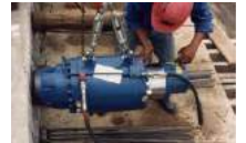
Gambar 6. Stressing Equipment
