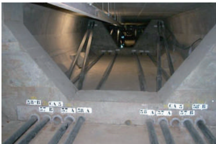
HDPE ducts for external prestressing
