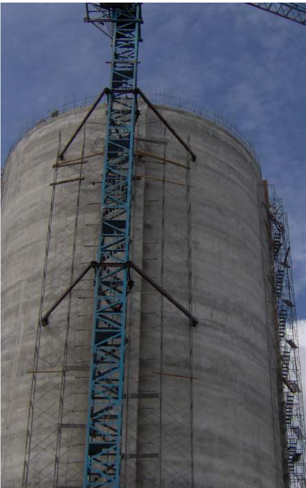
Post-tensioning Silo, Aceh
