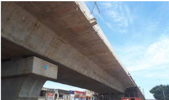
Flyover Simpang Susun Surabaya, Aceh
