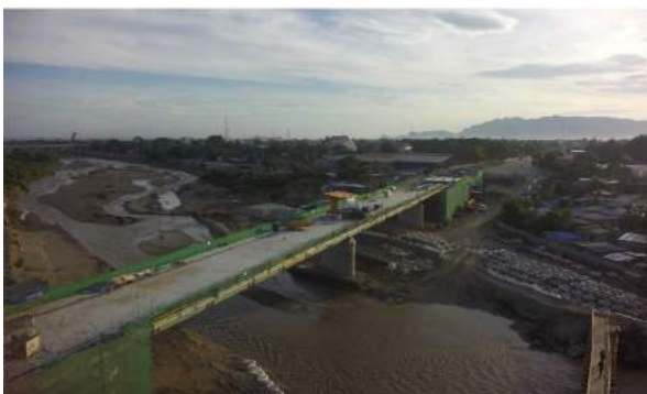
Comoro bridge, Timor Leste
