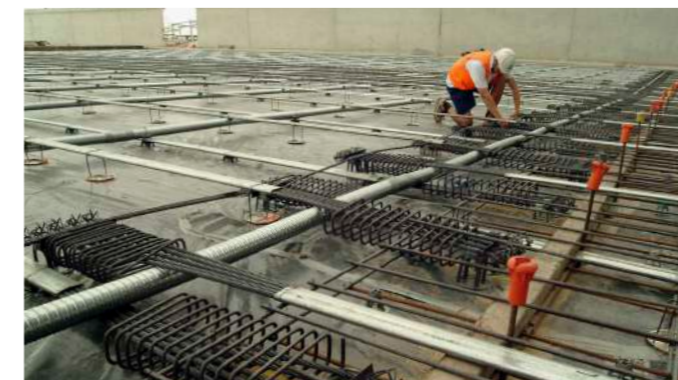
Townsville Sugar Terminal Australia | Post-tensioning bar systems
