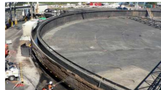
Curragh Mine Thickener Tank Australia | Repair
