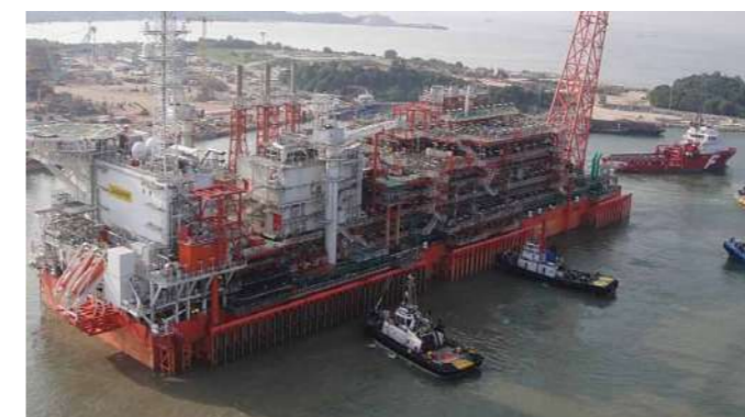
Jangkrik Complex Gas Extraction Indonesia | Bearings
