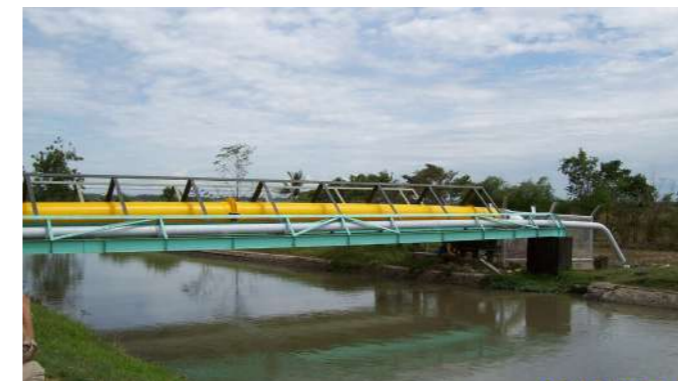
Pertamina Balongan Pipeline Indonesia | External Post-Tensioning
