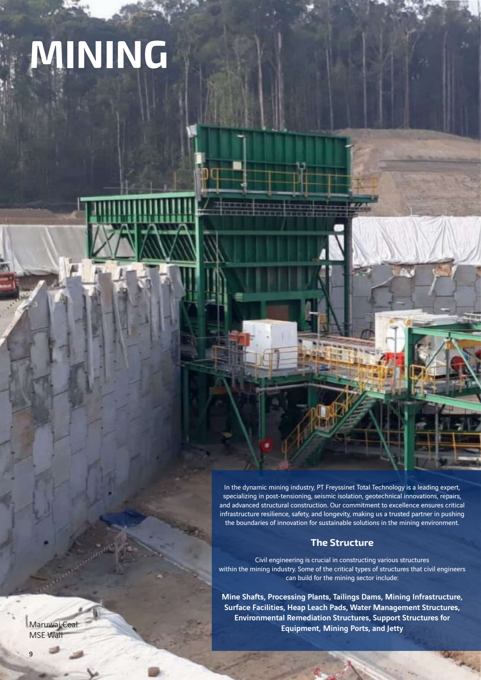
Martabe Gold Mine Indonesia | Reinforced Earth MSE Wall
