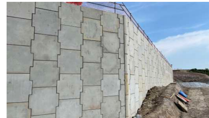
Martabe Gold Mine Indonesia | Reinforced Earth MSE Wall
