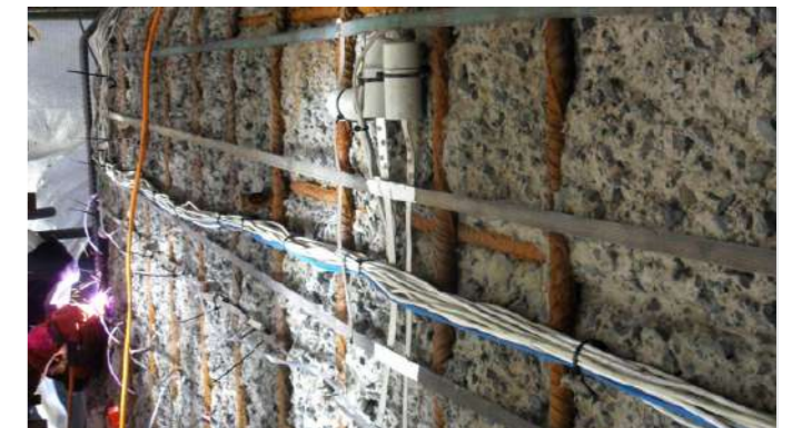
Kooragang & Carrington Coal Terminal Wharf Australia | Repair
