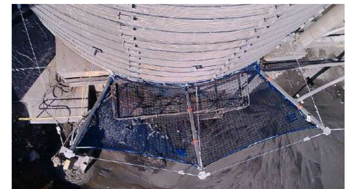
CSA Mine Cobar - Copper Ore Bin Remediation Australia | Repair
