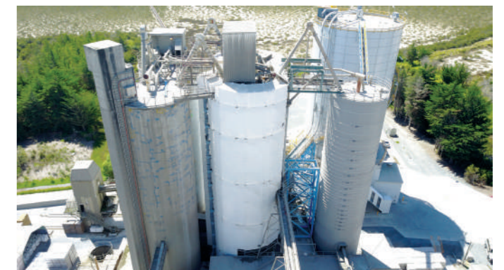
Golden Bay Cement Silo New Zealand | Repair and additional post-tensioning
