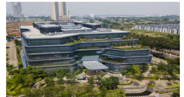
Unilever Indonesia Headquarter Indonesia | Post-tensioning bar systems
